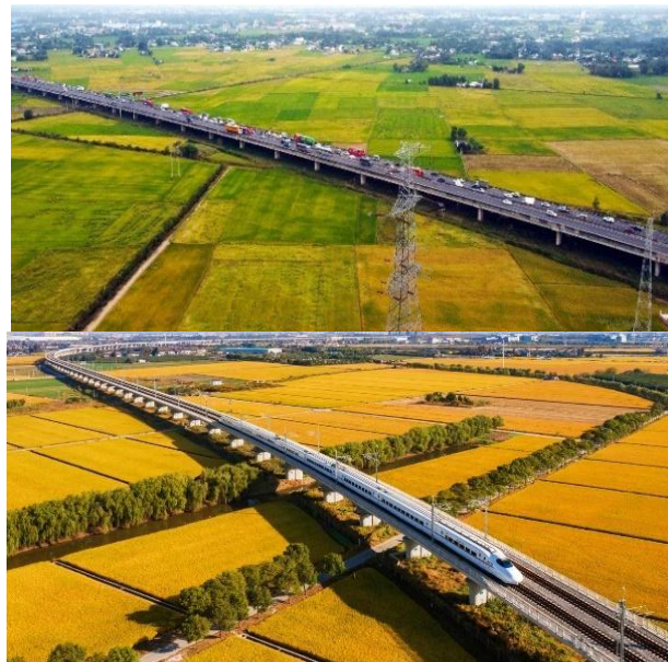
Figure 8.3: Full Excess Controlled Elevated Highways and Railways in Vietnam and China, Minimizing Ground Footprint
