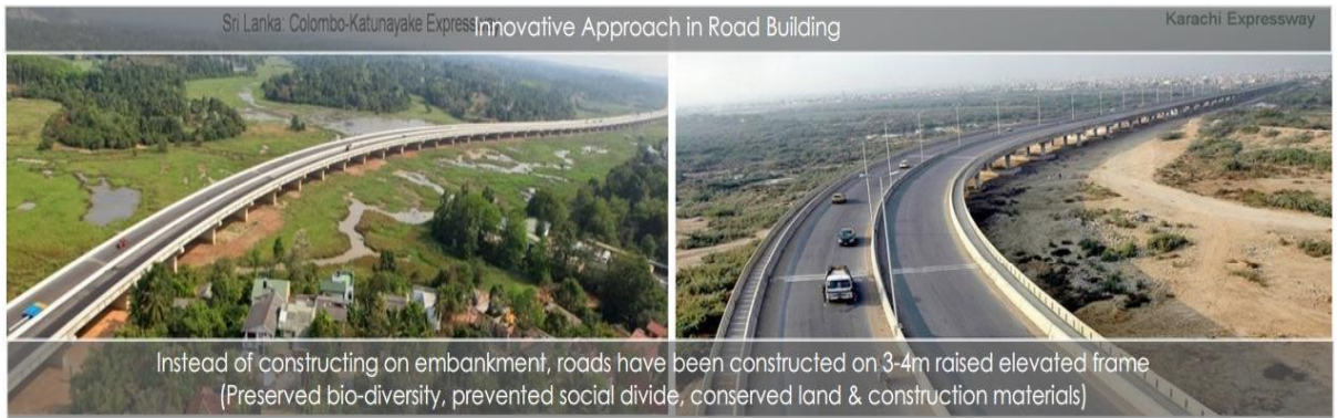
Figure 8.2: Land and Resource Conservation Potential Elevated Highways in Sri Lanka and Pakistan.
